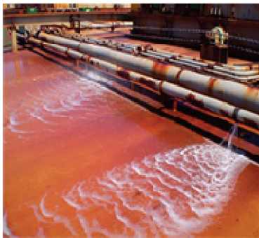
Holed fire line on deck
