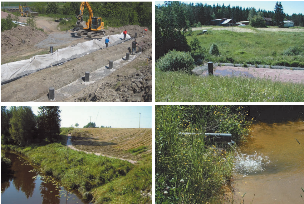
Figure 8. Experimental sand-filters of different structures and sizes are tested in the Pyhäjärvi catchment.
