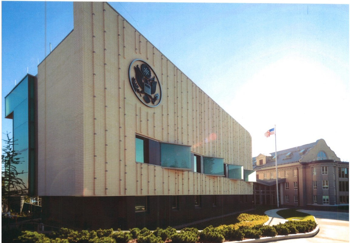
Figure 18 Finished consular building and Innovation Center
