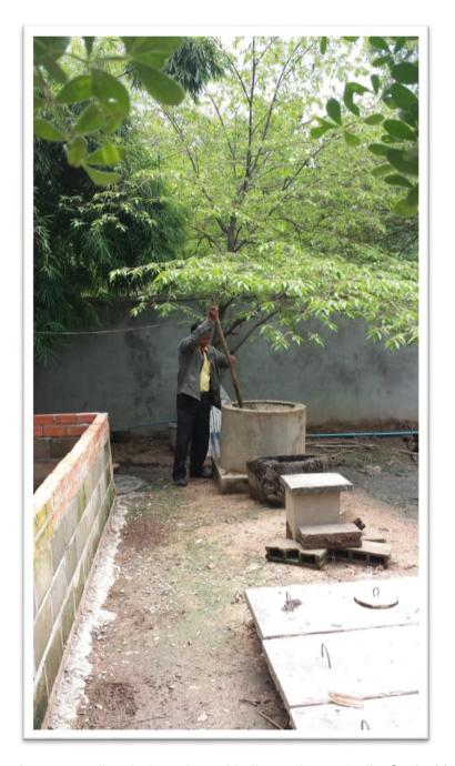
Picture 3 Feeding the input into a biodigester in Cambodia, © Visa Tuominen
