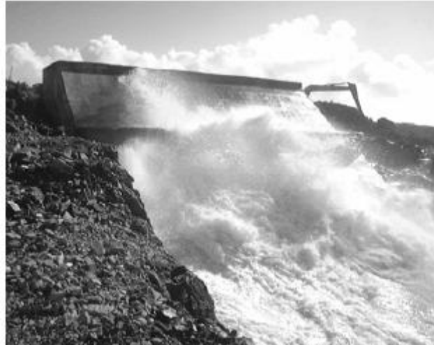
Figure 124. Shoreline-based Concrete Device in Scotland (WEC 2007).
