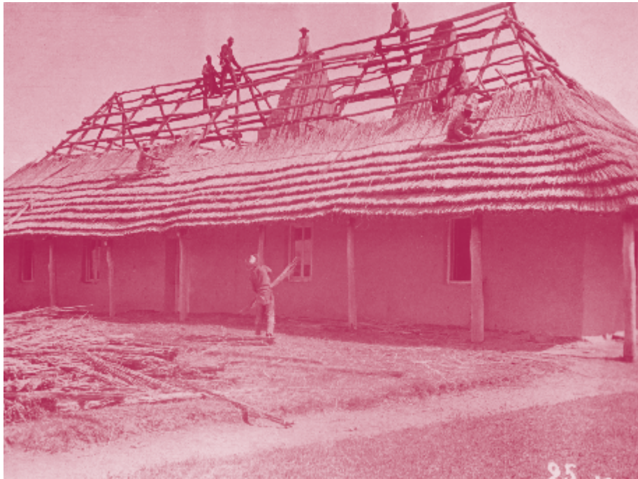
A new school building at the Ondangua station. The Finnish Heritage Agency. Photograph: Hannu Haahti (1911).
