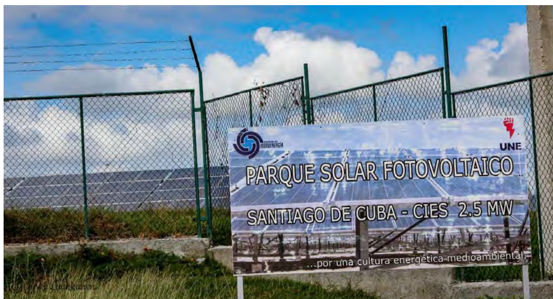
The solar power plant, Abel Santamaría
