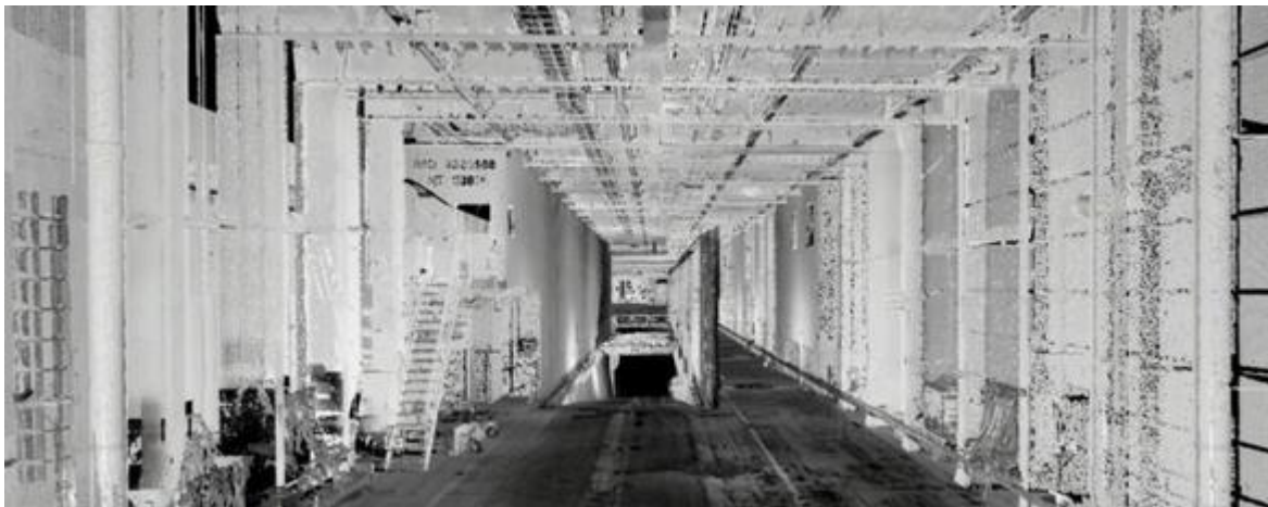
Figure 5 3D laser scanning of a DFDS vessel was carried out in collaboration with the Chalmers University of Technology (© Chalmers University of Technology)
