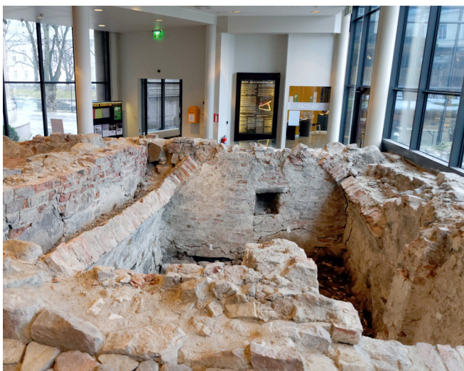
Figure 6. Cellar K92:6 in the entrance hall of Aboa Vetus & Ars Nova. The upper part of the walls and the barrel vault ceiling was made of bricks. The floor is paved with cobblestones, which are mainly rounded loose stones with the diameter of about 10–20 cm. Photo: Markus Kivistö.
