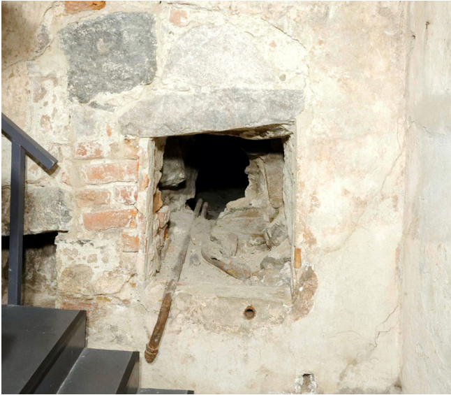
Figure 12. All analyzed stones can be found in the northeast corner of the cellar K93:4. The darkest stone on the left above the niche is mica gneiss - mica schist (type 2), the light-grey one next to it is quartz granite (type 2) and the one below it (above the opening) is hornblende granite (type 9). Photo: Markus Kivistö.
