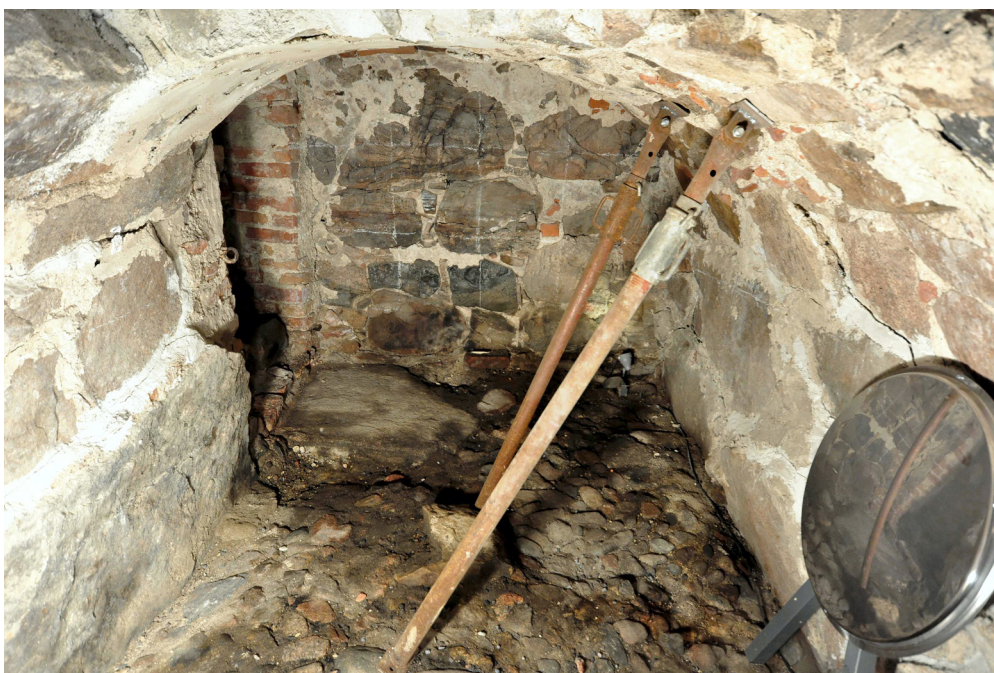
Figure 18. Cellar K95:21 was mainly made of dimension stones. The analyzed step stone can be seen in front of the back wall. Photo: Markus Kivistö.
