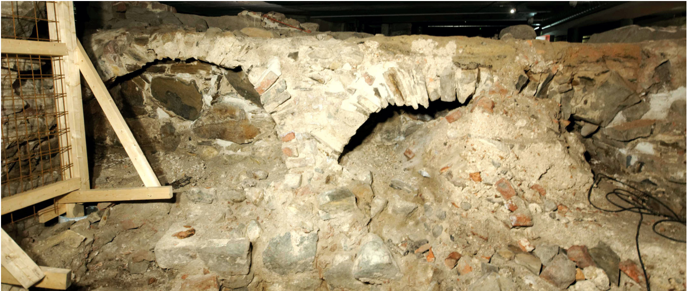
Figure 26. The southwest wall of cellar K94:9 with two arched recesses. The stones visible in the eastern recess on the left are all mica gneiss – mica schist (type 2). -At the time of this study, archaeological excavations in this cellar were still going on. Photo: Markus Kivistö.
