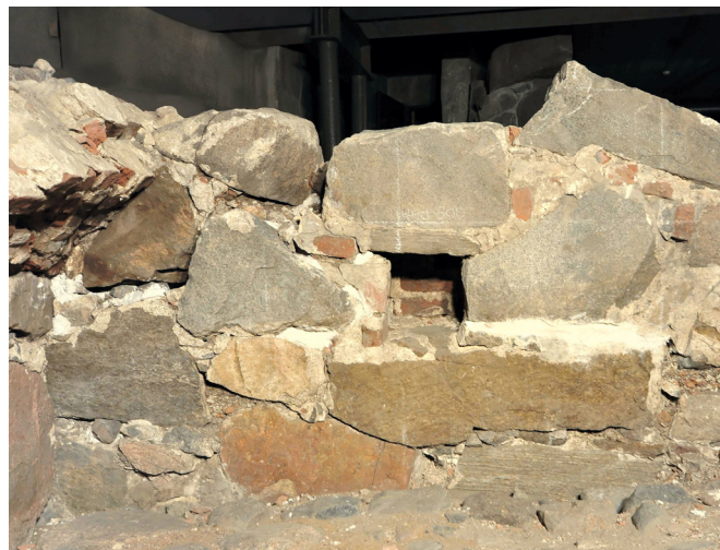
Figure 22. Some stones of notable sizes have been used in the south-west wall of cellar K94:12. From this wall nine stones were analyzed and they all can be seen in this picture. Three gray stones framing the niche are gradiorite (type 4), which is the most often used stone type in this cellar. The reddish one on the foot of the wall is quartz granite (type 1) and the big block below the niche is mica gneiss - mica schist (type 6) that are also frequently used in this cellar. Photo: Markus Kivistö.
