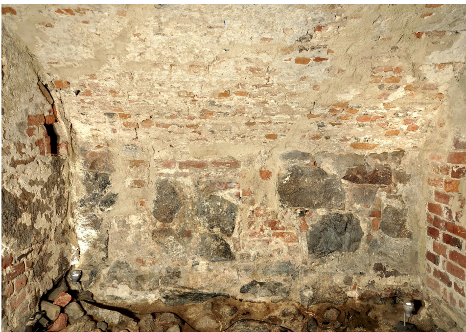
Figure 16. The cellar K93:3 was mainly made of bricks, but some stones were used in the northwestern (front) and northeastern (right) walls from where eight stones were analyzed and they represent all four stone types used in this cellar. Photo: Markus Kivistö.
