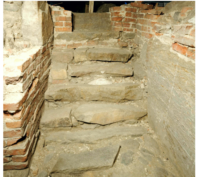
Figure 24. The stairs of cellar K94:11 are mainly made of quartz granite (type 1). The stepstone at the entrance leading to cellar K94:12 (on left) is mica gneiss – mica schist (type 2). The big block on the right side of the corridor is garnet cordierite mica gneiss (/kintzigite, type 8) which is is one of the biggest stones (1.2 m x 2.2 m) in the whole museum area. Photo: Markus Kivistö.
