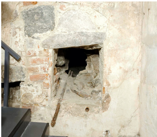
Figure 12. All analyzed stones can be found in the northeast corner of the cellar K93:4. The darkest stone on the left above the niche is mica gneiss - mica schist (type 2), the light-grey one next to it is quartz granite (type 2) and the one below it (above the opening) is hornblende granite (type 9). Photo: Markus Kivistö.
