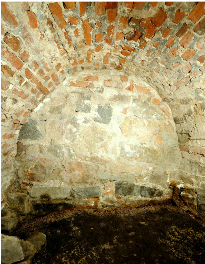
Figure 14. Cellar K93:5 was mainly made of bricks but stones were used in the northeastern wall and in the lower parts of the cellar. In this study, eight stones of this wall were analyzed. The dark grey one in the middle on top is the only quartz-feldspar gneiss (type 7) in this cellar. Photo: Markus Kivistö.
