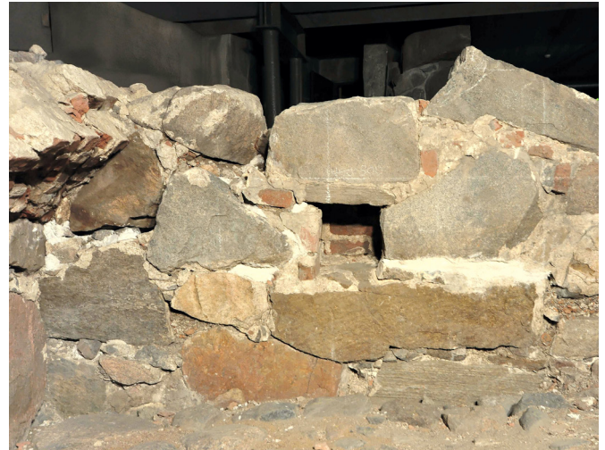
Figure 22. Some stones of notable sizes have been used in the south-west wall of cellar K94:12. From this wall nine stones were analyzed and they all can be seen in this picture. Three gray stones framing the niche are gradiorite (type 4), which is the most often used stone type in this cellar. The reddish one on the foot of the wall is quartz granite (type 1) and the big block below the niche is mica gneiss - mica schist (type 6) that are also frequently used in this cellar. Photo: Markus Kivistö.
