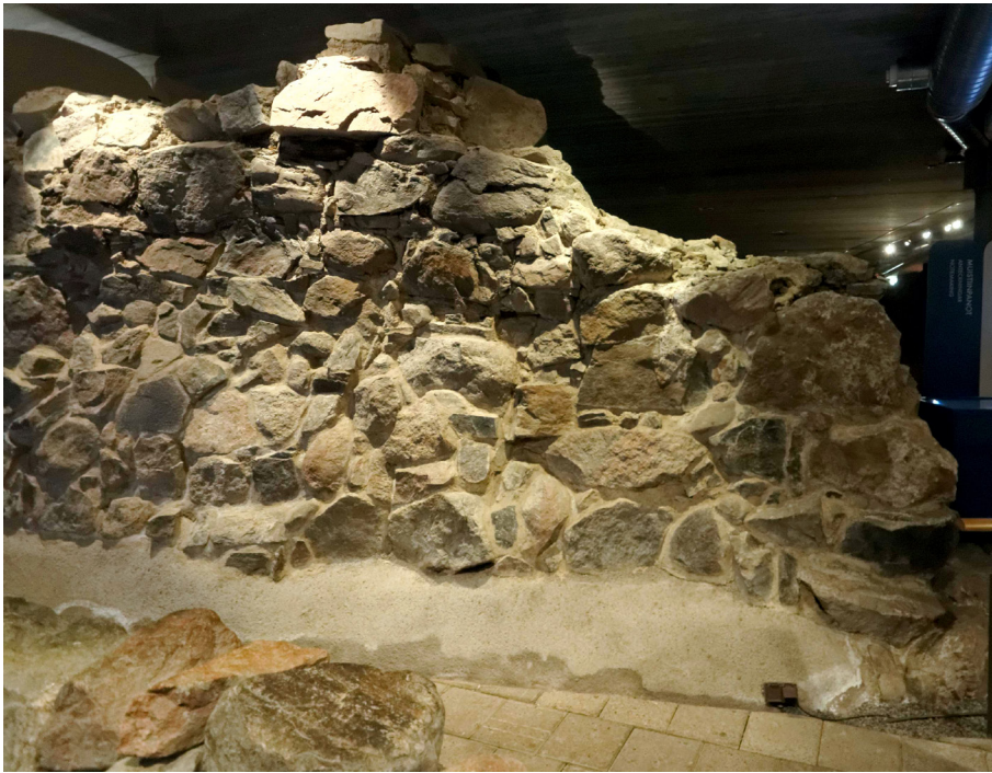
Figure 28. Even the largest stones in the northeast wall of the cellar K94:10 are round shaped suggesting that they can be loose stones (cf. K94:12). Therefore, only five stones from this wall were analyzed. The stones on the left below belong to a well that was not analyzed in this study. Photo: Markus Kivistö.
