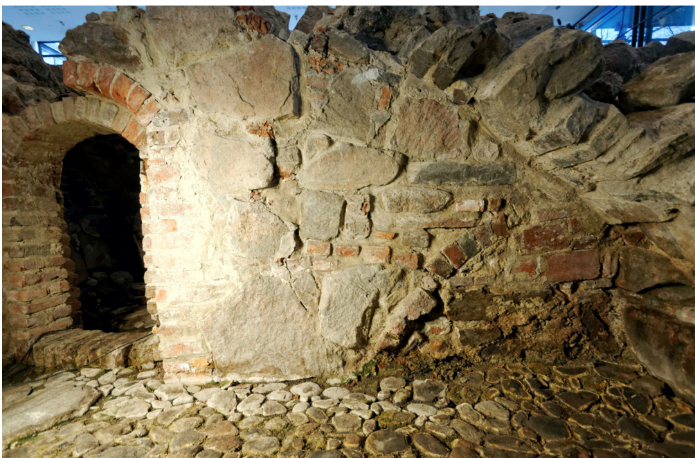
Figure 8. Six stones were analyzed from the northern wall of the cellar K92:3. The big block at the bottom of wall is the only red-black granite (type 6) among the analyzed stones in this context. The floor is paved with cobblestones (diameter about 10–20 cm), which were not analyzed in this study. Photo: Markus Kivistö.
