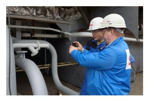
Fig. 1. Illustrative example of using a smartphone for augmented reality viewing of pipe installations. The system may e.g. present information about the purpose and material of individual pipes.
