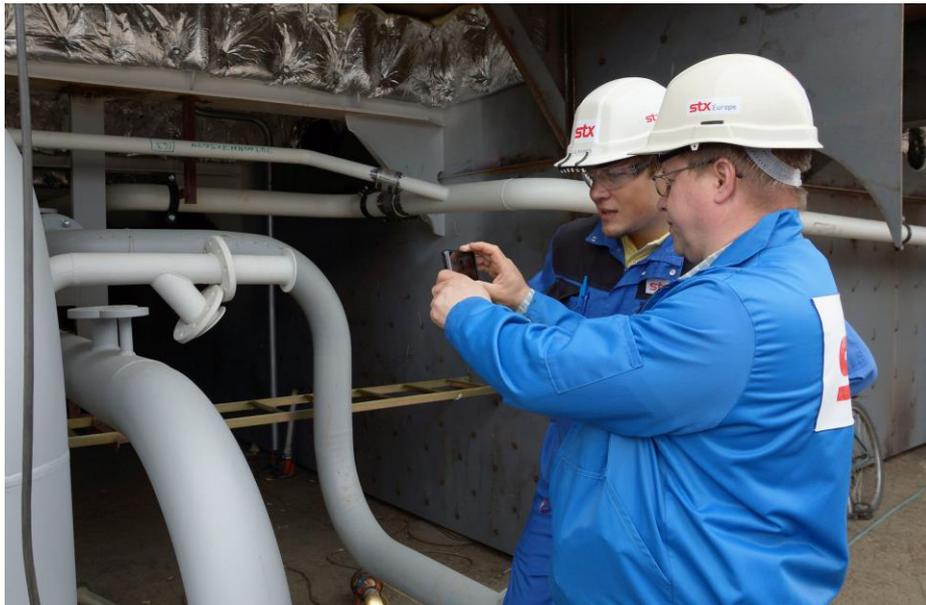
Fig. 1. Illustrative example of using a smartphone for augmented reality viewing of pipe installations. The system may e.g. present information about the purpose and material of individual pipes.
