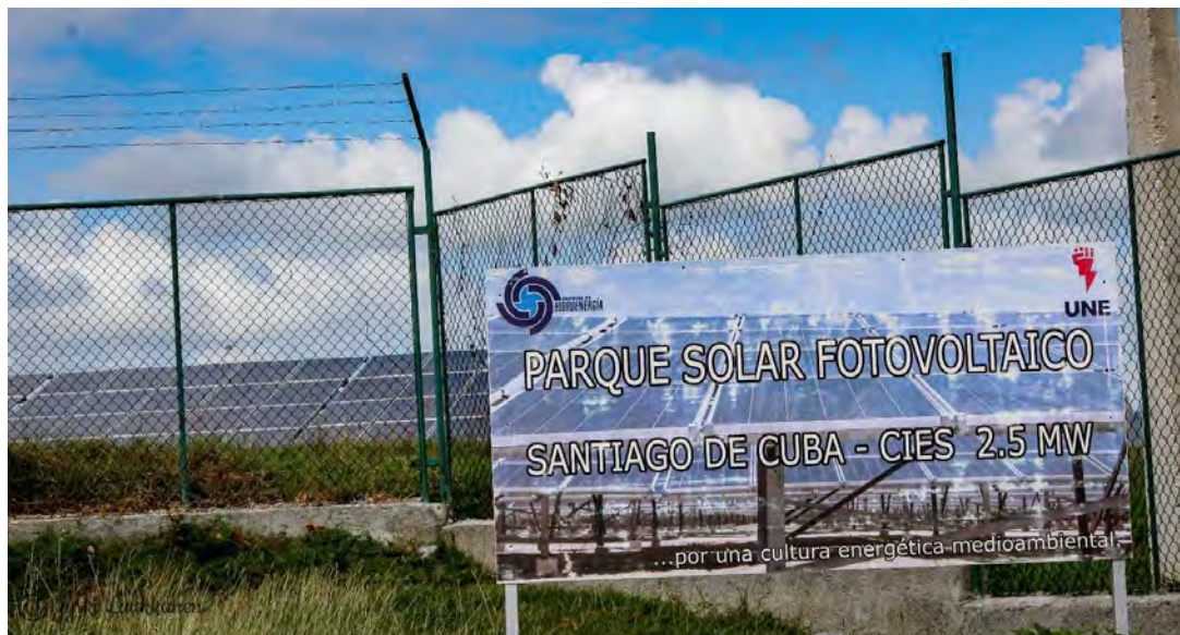
The solar power plant, Abel Santamaría
