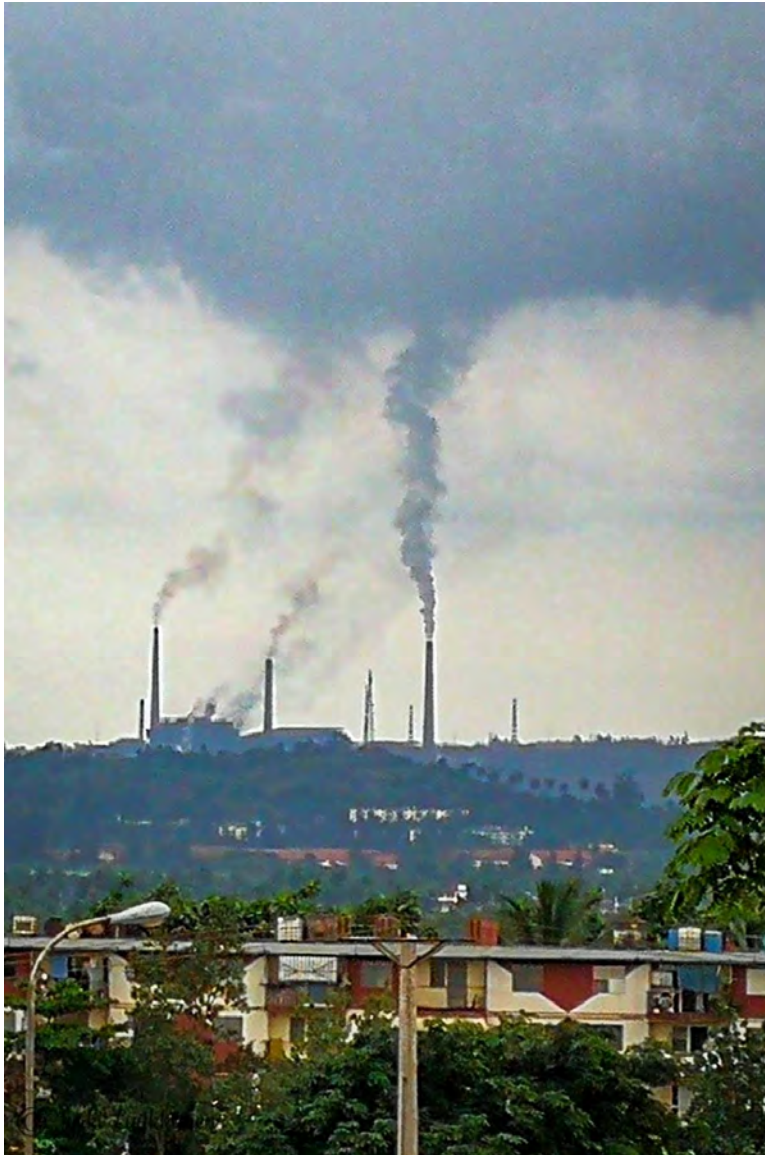
An industrial power plant, Moa
