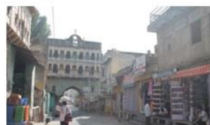
Darwaja-Sonthaliya Gate Gateways were built in different directions leading to main cities – only 20th century Sonthaliya gate survives
