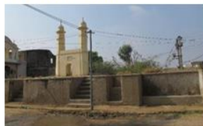
Historic water harvesting structures
