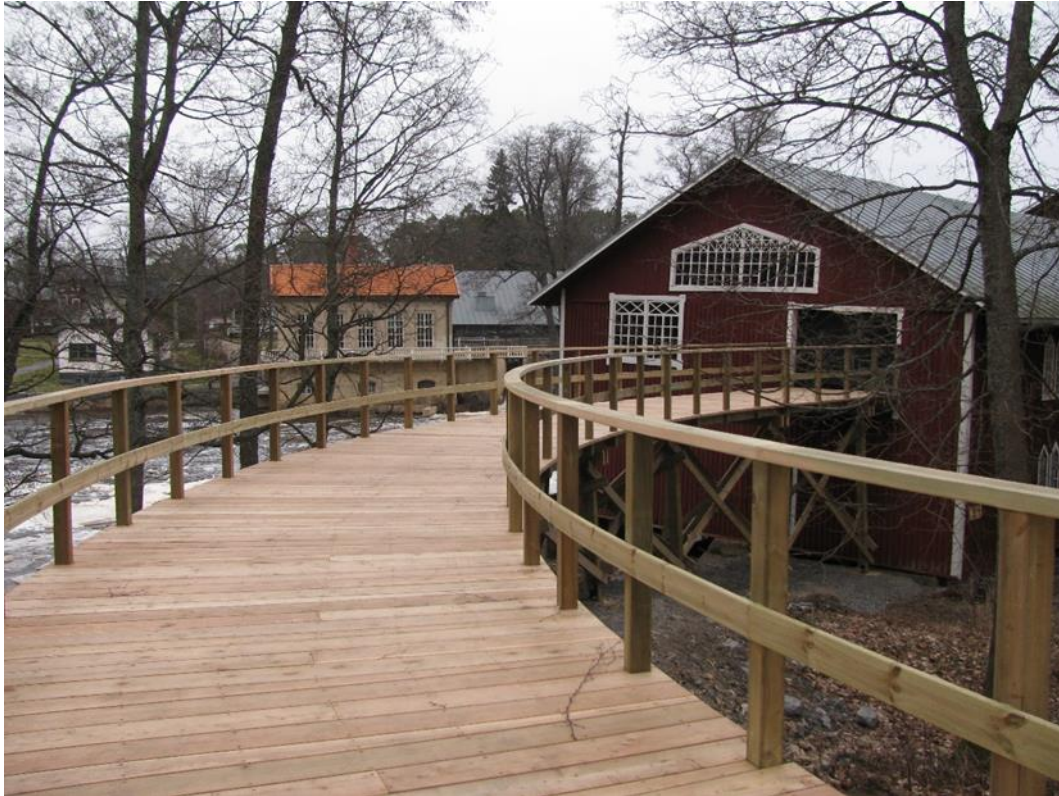
Figure 2. During the sawmill museum project, the architects got an inspiration from an old photograph taken in 1950's. A new bridge to the museum was constructed following the direction of the original rails that once led from the sawmill to the timber yard (Photo: Grahn, 2014).
