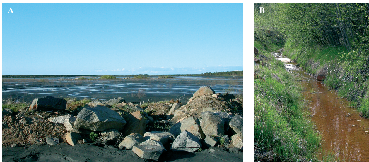
Fig. 3. a) Overview of the Hitura tailings area seen from south in 2004. Disposal area “C” in the front (Photo: Paola Frattini). b) Seepage collection ditch surrounding the Hitura tailings area (Photo: Päivi M. Heikkinen).
