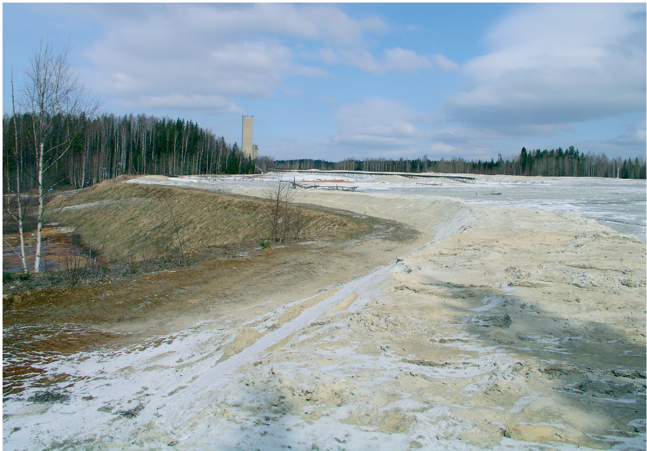
Fig. 5. The Luikonlahti tailings area with magnesite tailings covering sulphide tailings in spring 2005. The upper section of the constructed dam is seen on left (Photo: Marja L. Räisänen).
