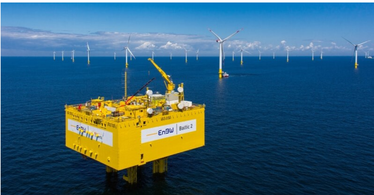
Figure 1 Substation platform at the Baltic Sea 2 offshore wind site. (Froese, 2016)
