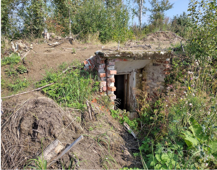
Figure 2. A German-built cellar in Pori after it had already been run over by excavators. Soon after, the construction was demolished and covered with sand. Photo: Teemu Väisänen.
