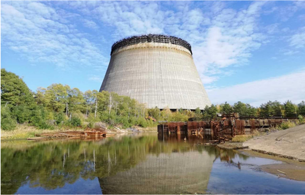
Figure 2. Unfinished cooling tower in the CEZ. Photograph taken in October 2019 by Veera Ojala.
