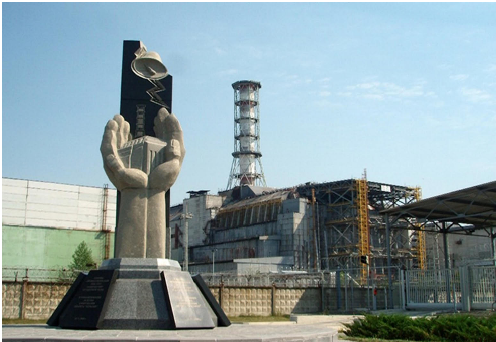
Figure 28. The nuclear power plant covered by a Soviet built sarcophagus in 2008. Source: Jim Hart, reproduced with the author's permission.
