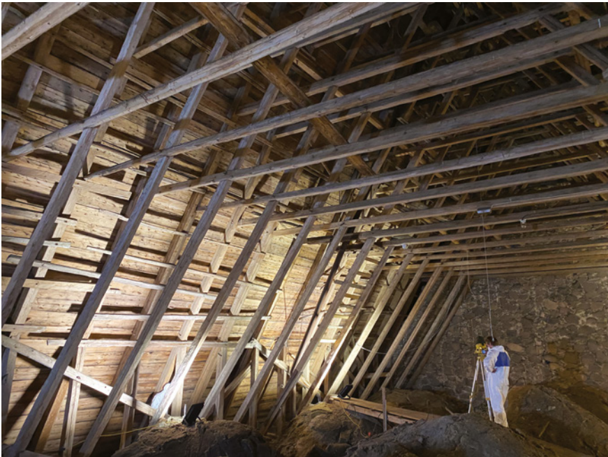
FIGURE 5 The roof structure of Pyhtää church (1461–1462d) PHOTO: PANU SAVOLAINEN
