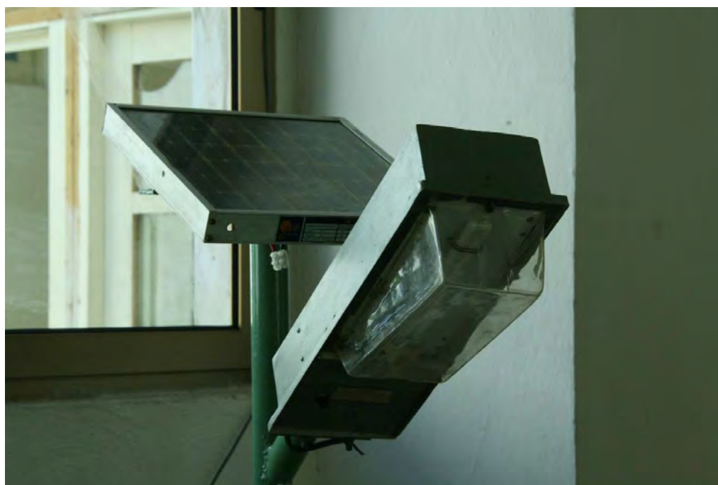
Street lighting with a photovoltaic panel
