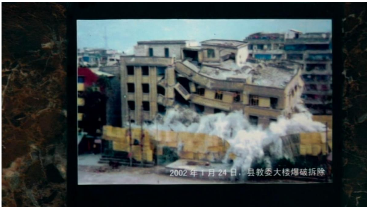
Figure 9. 58:02. Photo of a building being demolished. 2002年1月24日，县教委大楼爆破拆除 (2002 nián 1 yuè 24 rì, xiàn jiàowěi dàlóu bàopò chāichú, "On January 24, 2002, the County Education Commission building was demolished by blasting").
