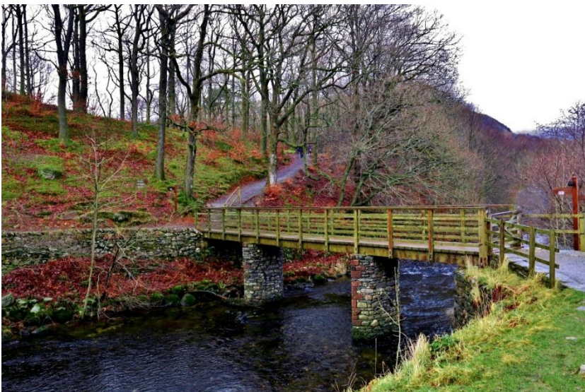
Figure 41. Old bridge in the wilds.
