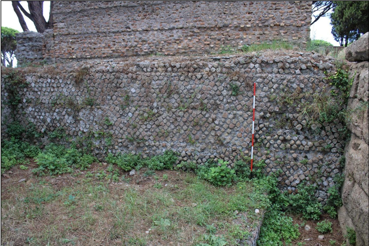
Figure 5: A section of the city walls between the Porta Laurentina gate (on the right) and its western tower in Parco Archeologico di Ostia Antica. The facing of the walls in opus quasi reticulatum is attested, but according to the stratigraphic analysis by Glogowski (2023: 116–120, 128) only the part in the lower right corner, with a more eroded appearance, is original structure. The rest of the wall is either ancient or modern restoration, with Glogowski inclining towards the latter option. Behind and above the walls are the remains of the temple of Bellona. From south-east. Picture by author.
