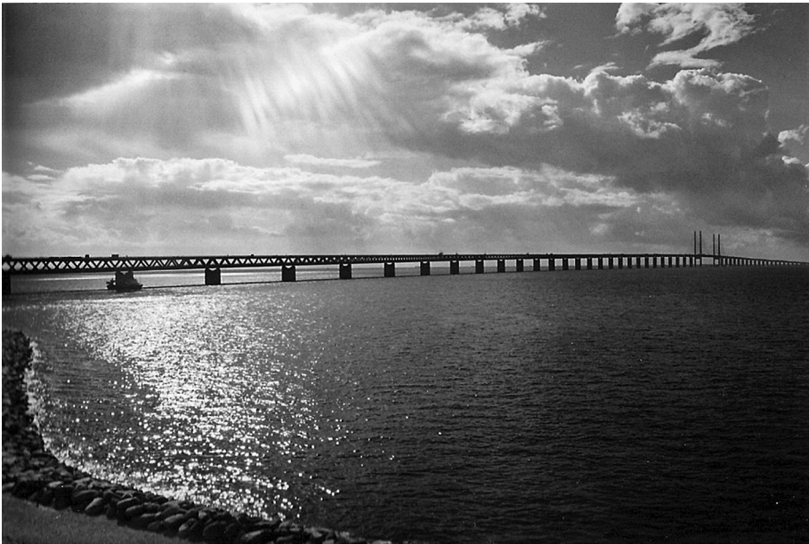
Figure 7. The Øresund Bridge under construction in 1999. Malmö, Sweden, Kiiskinen.
