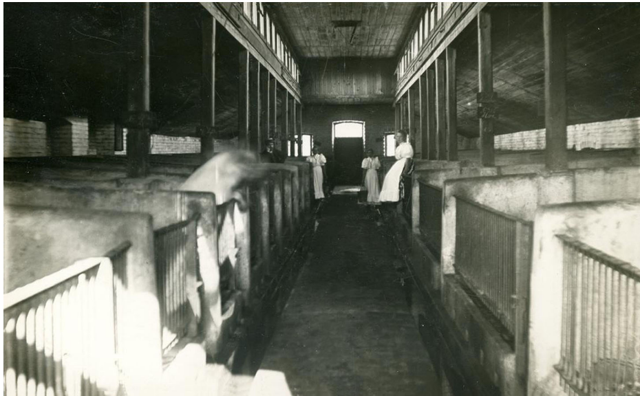
FIGURE 1. A modern piggyery with concrete pen walls at Vuojoki Mansion in western Finland in 1905. Johan Ludvig Nordberg, Rauma Museum, Rauma Museum photographic collections (RMK117).
