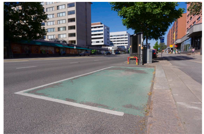
Fig. 4. A charging area marked in green. Photograph: author / CC BY 4.0.
