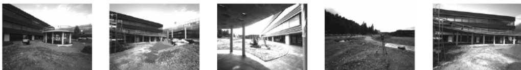
Figure 3.2: Hilti Construction Site Outdoor 1
